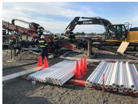
Horizontal well installation in 2017
